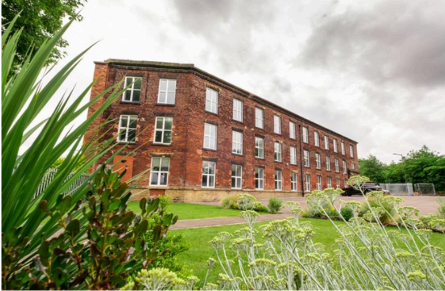
Albion Court, Bolton, Greater Manchester
