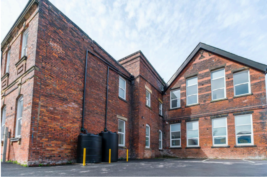
St Mary's Court, Preston, Lancashire
