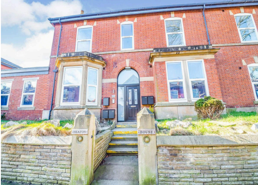
Heaton House, Bury, Greater Manchester
